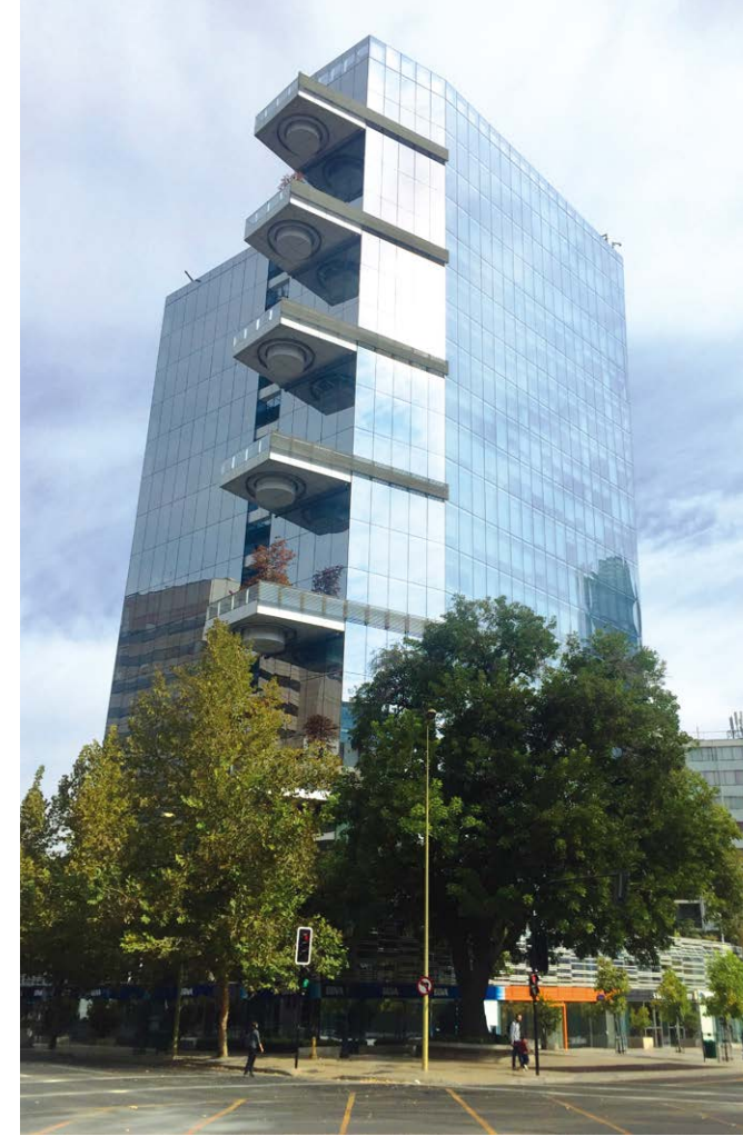
Territoria El Bosque LEED Certified · Santiago, Chile · Commercial Building · Product: Multi V III Heat recovery
