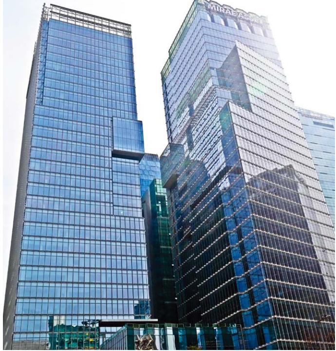
Mirae Asset Center 1 LEED Silver · Seoul, Korea · Commercial Building · Product: Multi V Water II, Chiller
