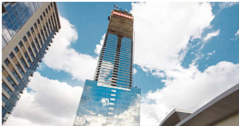
KOI Project LEED Silver · Monterrey, Mexico · Commercial Building · Product: Product: Multi V Water IV
