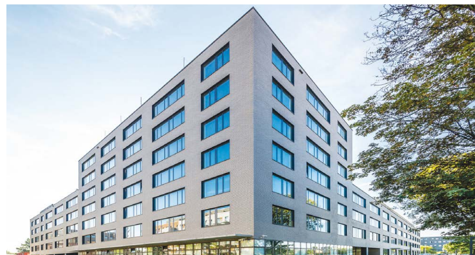
Promenade ZITA LEED Platinum · Wrocław, Poland · Commercial Building · Product: Multi V IV Heat recovery
