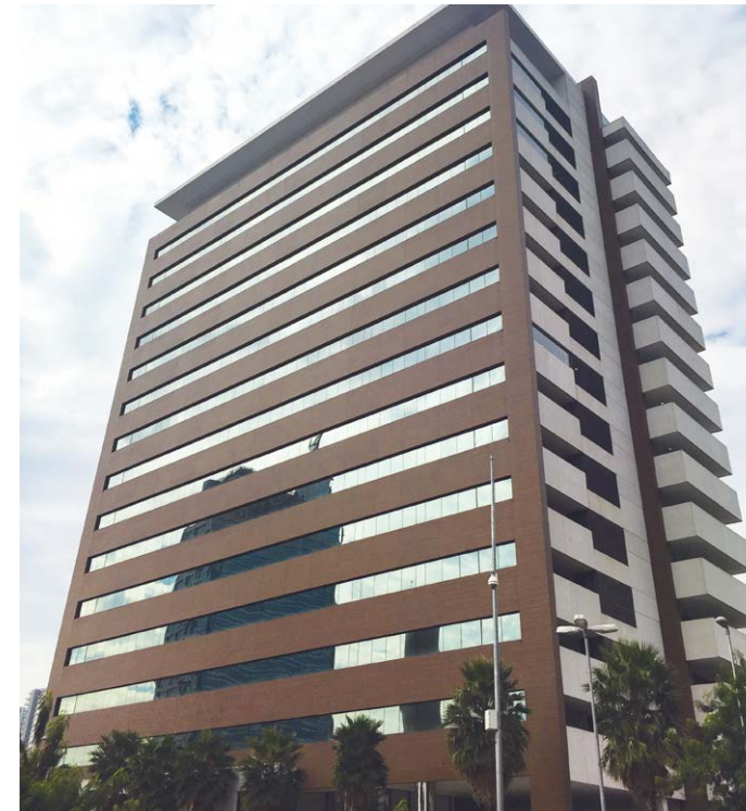
Edifício Grand Station LEED Gold · São Paulo, Brazil · Commercial Building · Product: Multi V III
