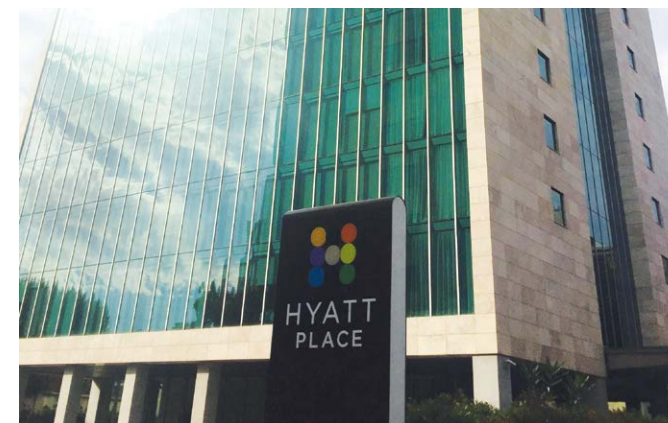
Hotel Hyatt Place LEED Certified · Santiago, Chile · Accommodation Facilities · Product: Multi V Water Heat recovery
