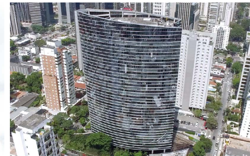
Infinity Tower LEED Gold · São Paulo, Brazil · Commercial Building · Product: Multi V Water II
